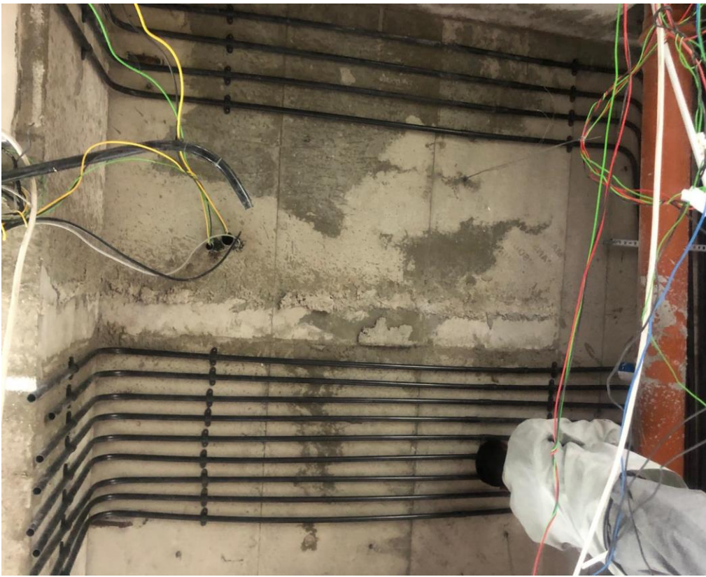
Electrical Conduiting works
