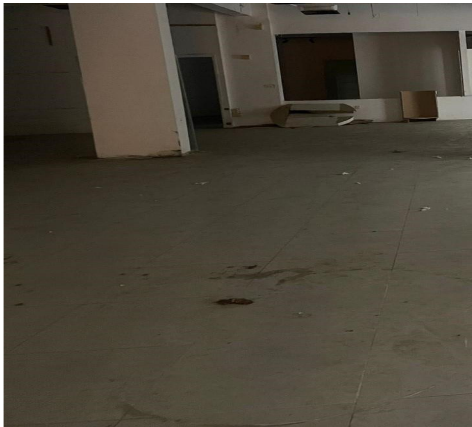
Stores Full Renovation
